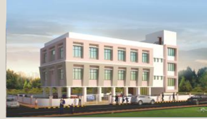
COMMUNITY CENTER - GHANSOLI
