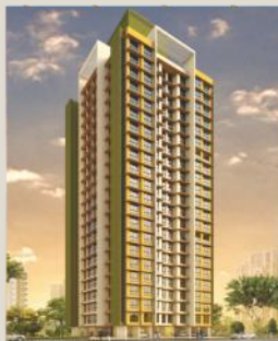
ADITYARAJ AVENUE VIKHROLI
