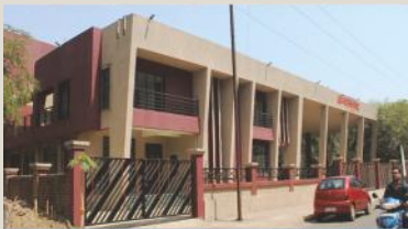
FIRE STATION - KOPERKHAIRANE
