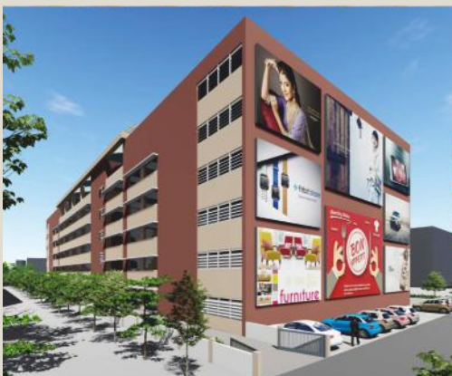
PARKING TOWER BUILDING CBD BELAPUR
